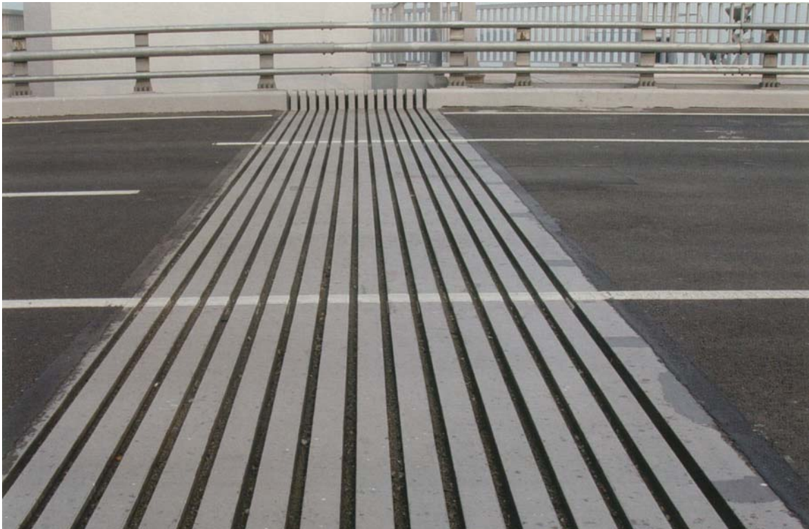
Installed 15 seal MAURER Swivel Joist Expansion Joint DS 1200
